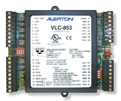
The Alerton® BACtalk® VLC-853 is a versatile, high-performance BACnet-compliant field controller designed for control of central plant systems, air handling units, large terminal units, and similar control and process equipment. As a native BACnet controller, the VLC-853 integrates seamlessly with your BACnet system. It communicates at up to 76.8 Kbps on a BACnet MS/TP LAN or can operate as a stand-alone controller.
